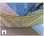
Place film on second section (partly overlap on first section)
